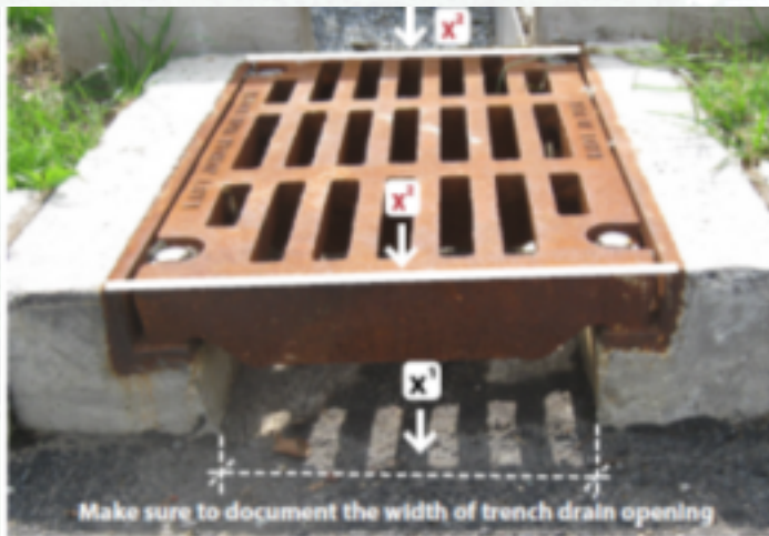
Trench drain: lowest point of trench drain, top of grate, and width of the grate.
