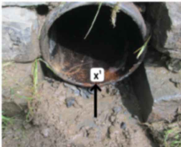
Pipe invert: bottom interior elevation of pipe
