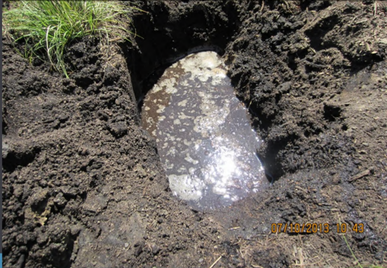
Failure 2: Flat geotextile created 'perched watertable'
