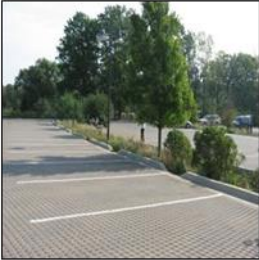
Permeable Pavement allows rain to infiltrate back into the ground.
