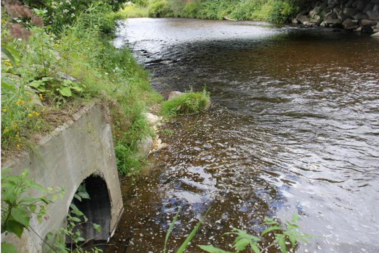
Combined Sewer Overflow
