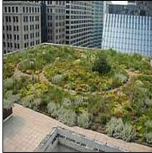
Green Roofs capture rain and save energy by cooling buildings.
