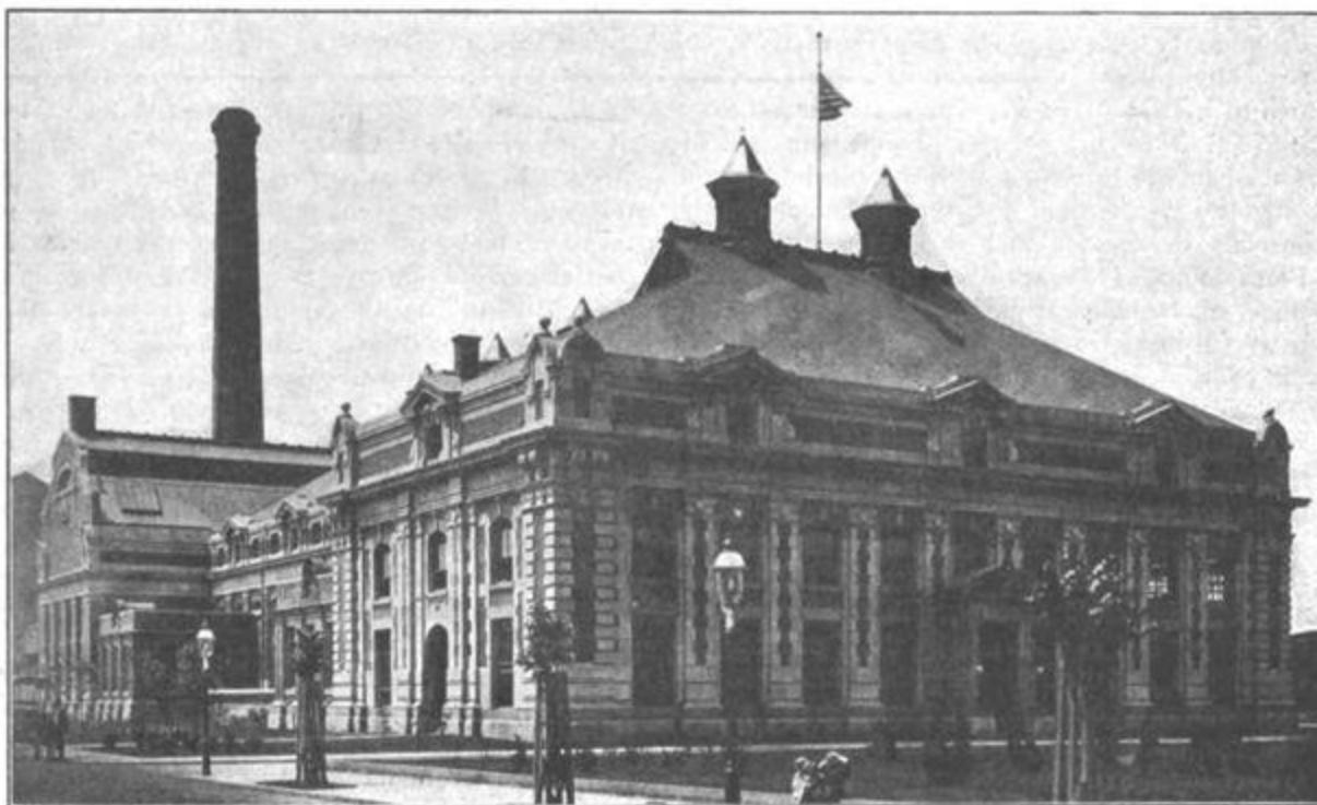
The New Sewage Pumping Station at Washington, D. C.
