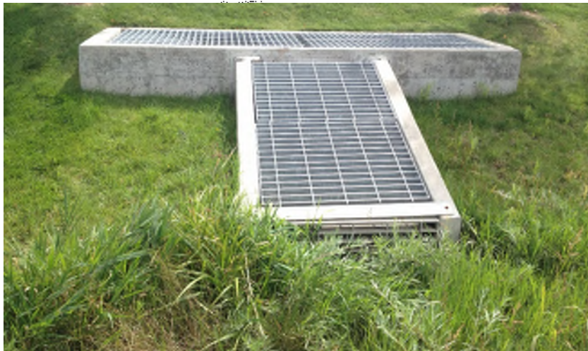
WATER QUALITY BASIN OUTLET STRUCTURE (CS-103)
