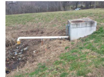
Structure is in good shape.
