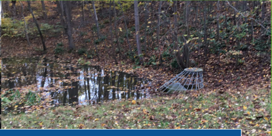
Before - Low flow is clogged, silted in & wooded
