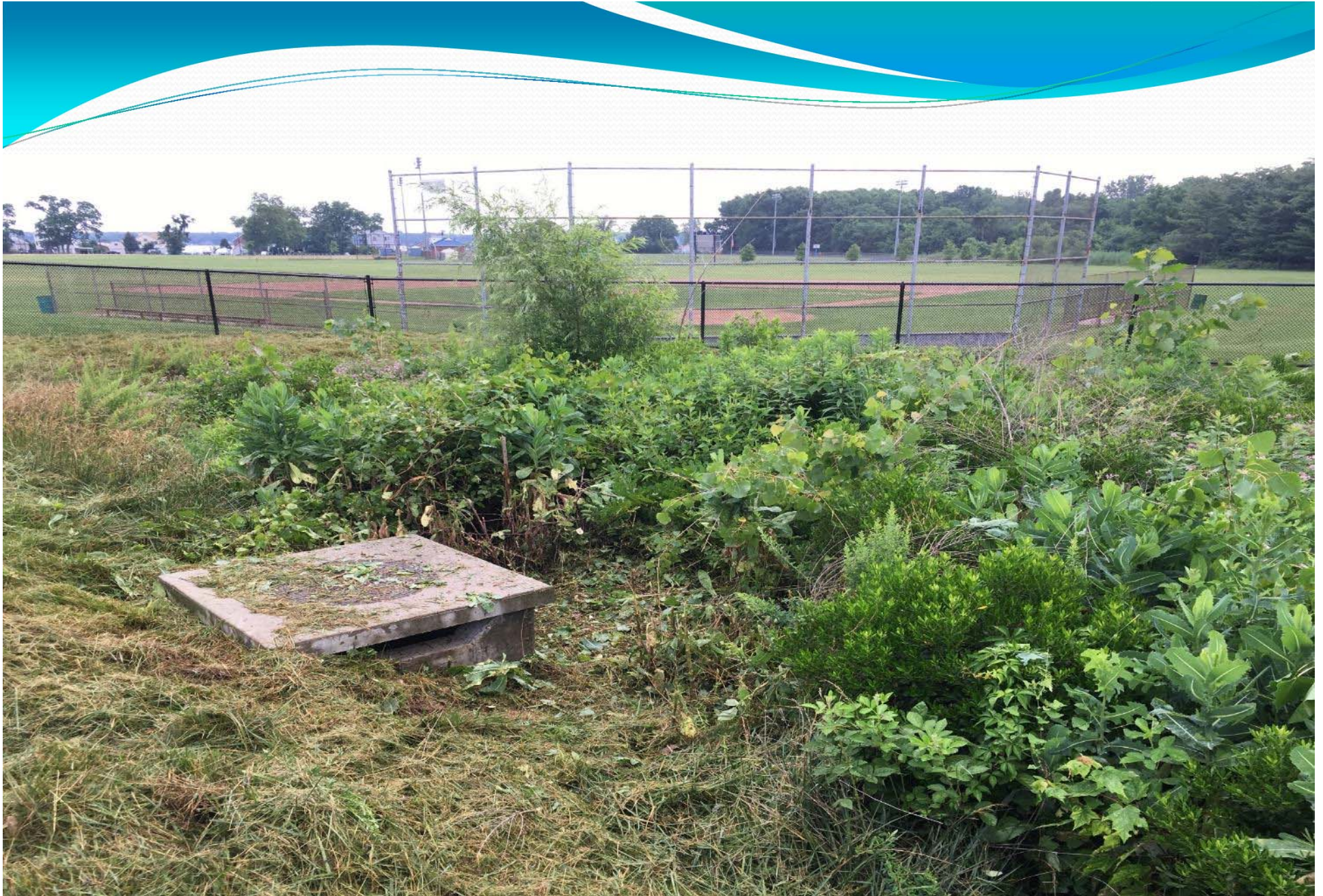
Sparrows Point Middle & High Schools-Facility 9.1
