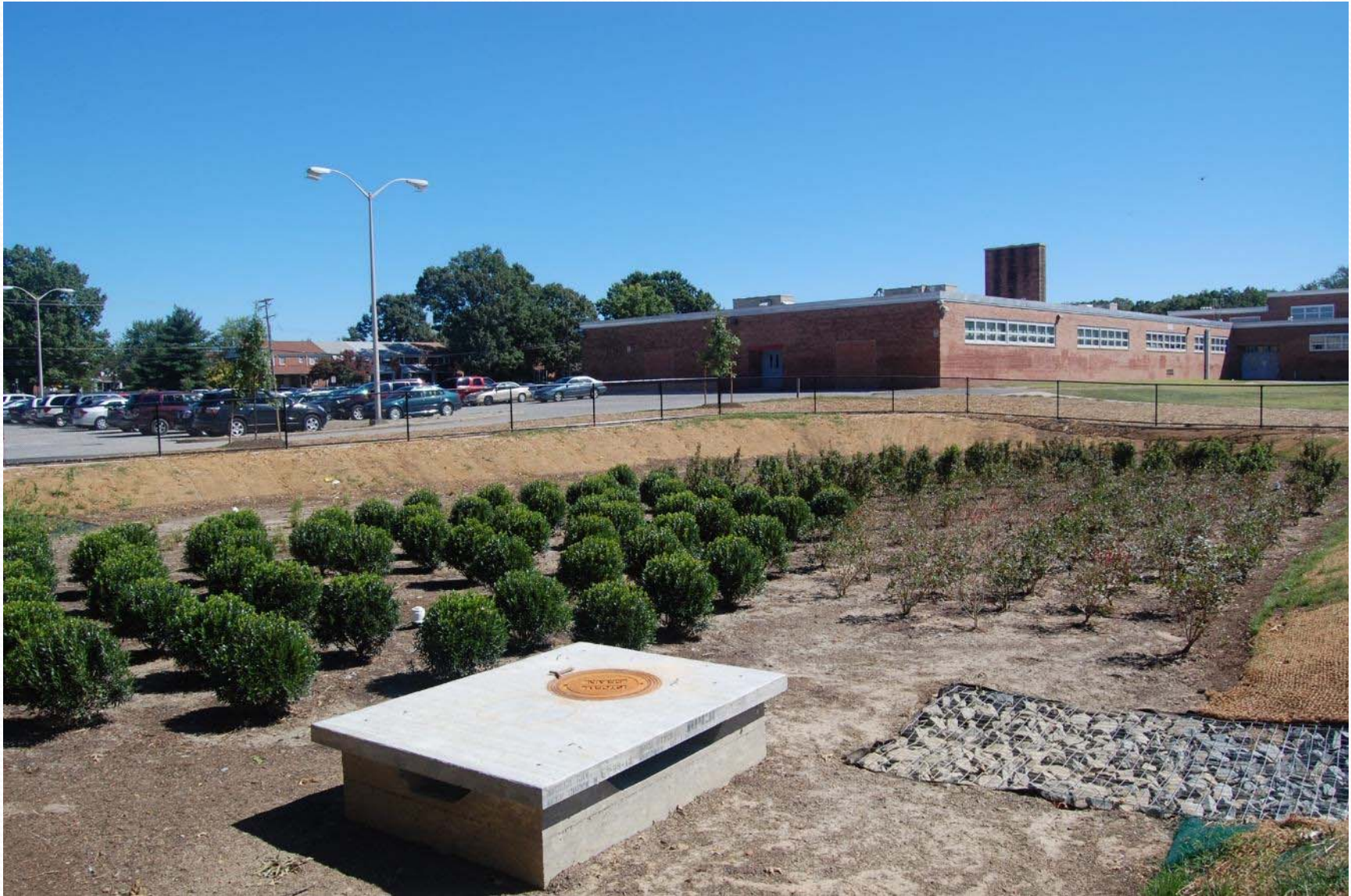
Deep Creek Middle School-Facility 6.1
