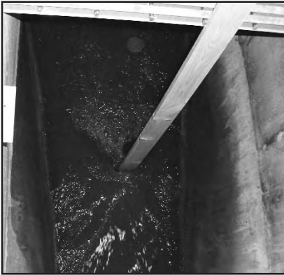
Figure 3: Maguire Group’s temporary energy dissipater
