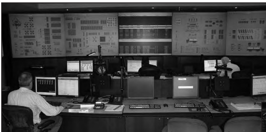
Left, Central Control Room. Five large screens on back wall are, from left to right: Primary/Secondary Treatment, Nitrification/Multi-Media Filtration, Alarms, Thickening/Dewatering, and Solids Processing.
