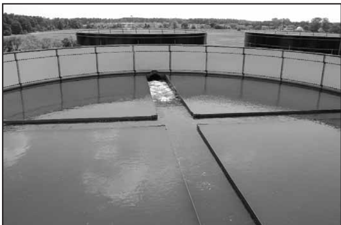
To Surface of Anoxic Filter Showing Effluent Trough
