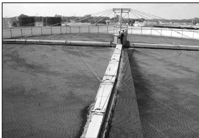
Top Surface of Oxidic Filter Showing Rotary Distributor Arms
