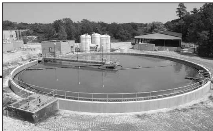
Primary Clarifier with 3 Storage Tanks for Ferric Chloride and Polymer
