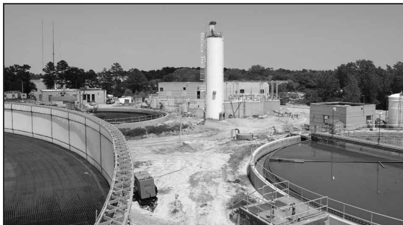
Lime Silo with Primary Clarifier on Right and Oxidic Filter on Left
