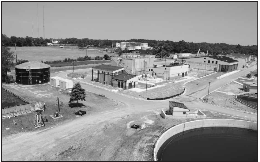
Rectangular Concrete Structure is the Final Effluent Denitrification Sand Filter
