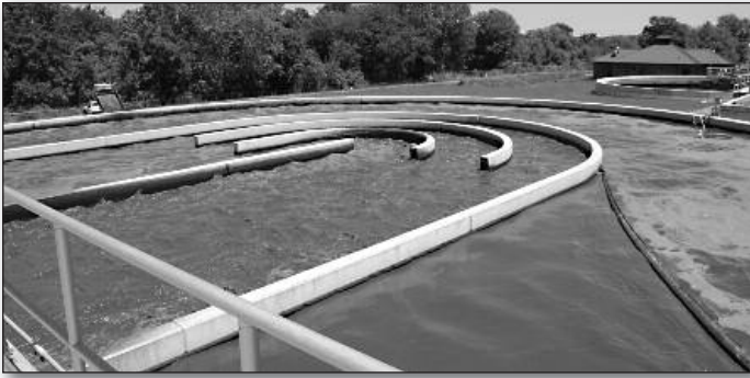
Bardenpho Reactor Tank
