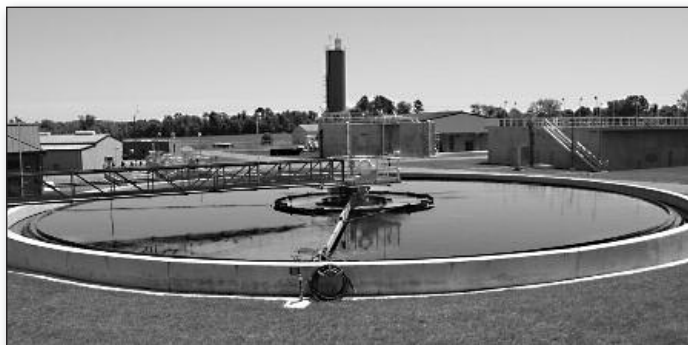
Secondary Clarifier with Class A Storage Silo in Background
