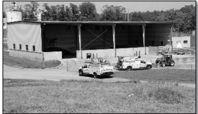
Biosolids Storage Building. Lime Silo is in Background.
