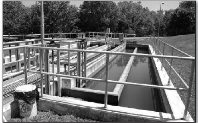
Chlorine Contact Tank
