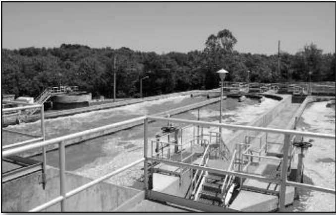
Bardenpho Carousel Reactor. Second stage of Bardenpho process. Gravity sludge thickener is shown in left background.
