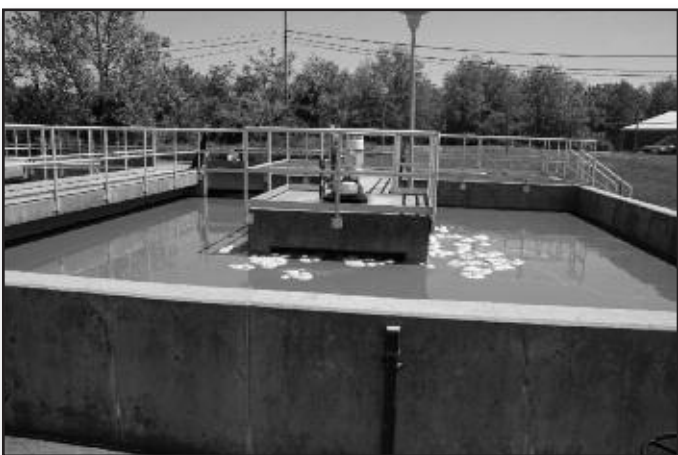
Second Anoxic Zone, Third stage of Bardenpho process.
