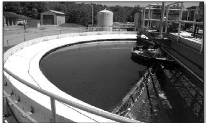
Secondary Clarifier, showing covers over weirs for algae control and liquid polyaluminum tank for phosphorus control in background.
