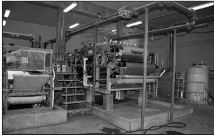
Two Belt Filter Presses
