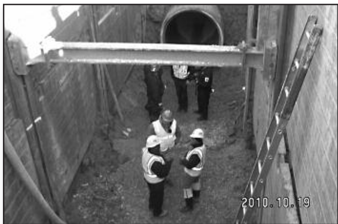
Dundalk Water Main Restoration—Kishia is on the right in the foreground
