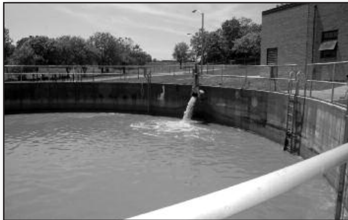
Equalization Basin At Head of Plant
