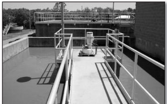
Anoxic Zone. First stage of Bardenpho process.
