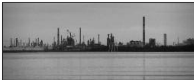
Refineries at Delaware City. Who says this country does not do much manufacturing?
