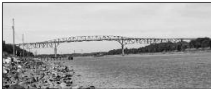
Reedy Point Bridge over Chesapeake and Delaware Canal near the canal’s eastern terminus.
