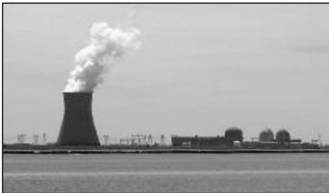
Hope Creek–Salem, New Jersey nuclear power plant.
