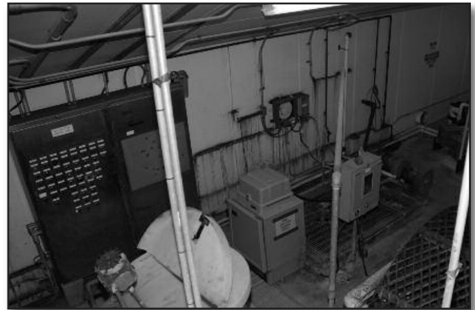
Plant Main Control Panel
