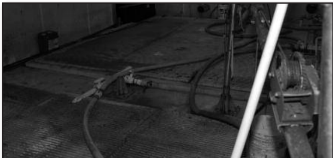
Grates Over Two Aeration Tanks
