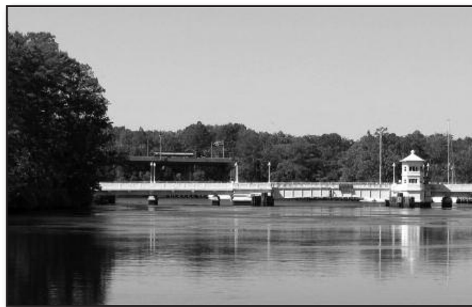
Market Street Bridge with Rt.13 bridge behind.
