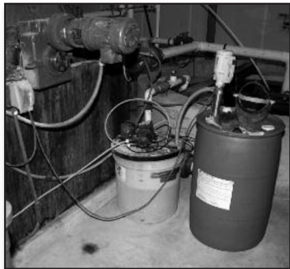
Liquid Coagulant Addition Equipment
