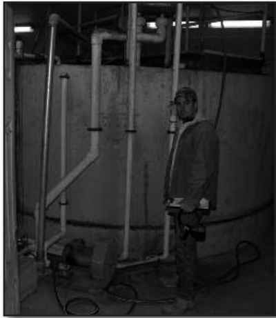
Side View of Former Primary Clarifier Now Used as a Reactor Clarifier
