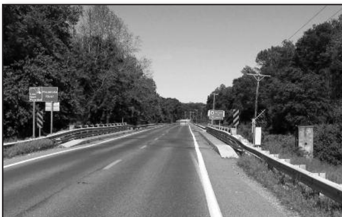
USGS gauging station (right side of guardrail) at Willards, Md.
