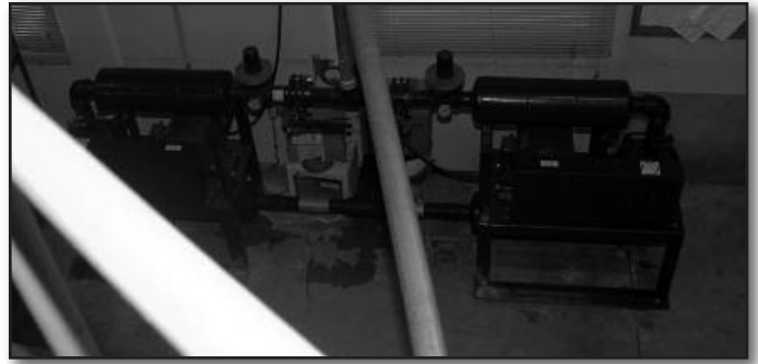
Two Blowers for Activated Sludge Process
