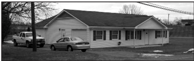
Single Story Ranch House Building Which Houses the WWTP
